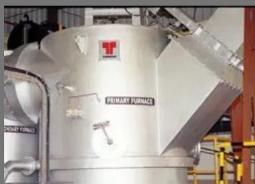
Thermax Solid Waste Incinerator
