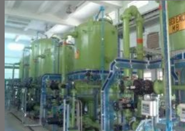
Thermax Commercial Water Softener Plant
